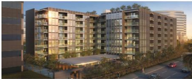
Next in line: 150-unit IBC complex planned near Century Centre offices
