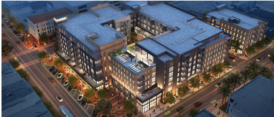
4th & Main: pair of 7-story residential towers planned in downtown Santa Ana
